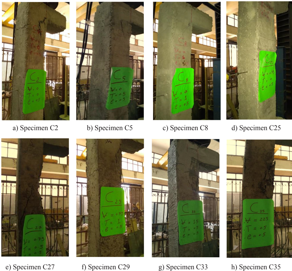
Fig. 5. Crack pattern and failure of columns tested under eccentric loads, eccentricity ratio, e/t = 0.50 .
